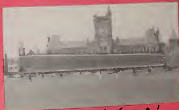
Tower Gone! No problems!
